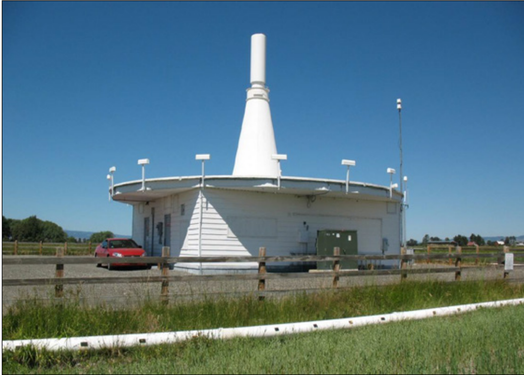
Figure 6-27. Enroute VHF Omnidirectional Range (VOR) facility
