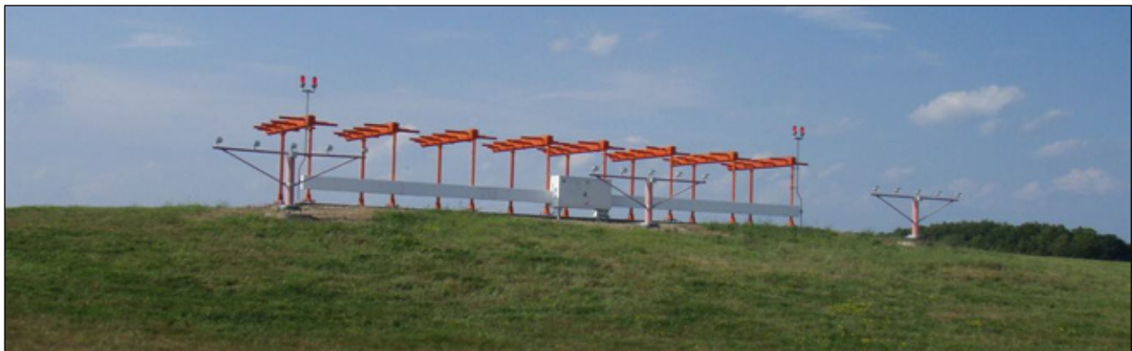
Figure 6-21. LOC 8-antenna array
