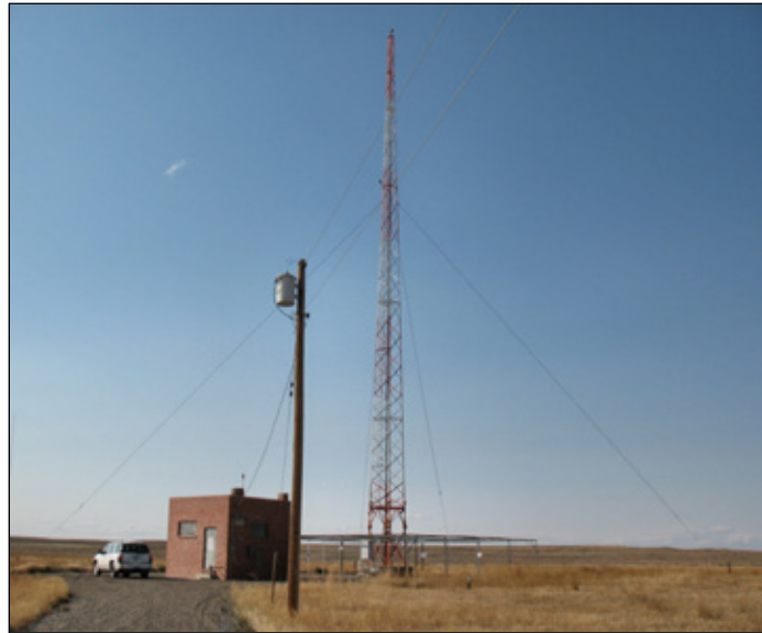
Figure 6-31. Non-Directional Beacon (NDB) facility
