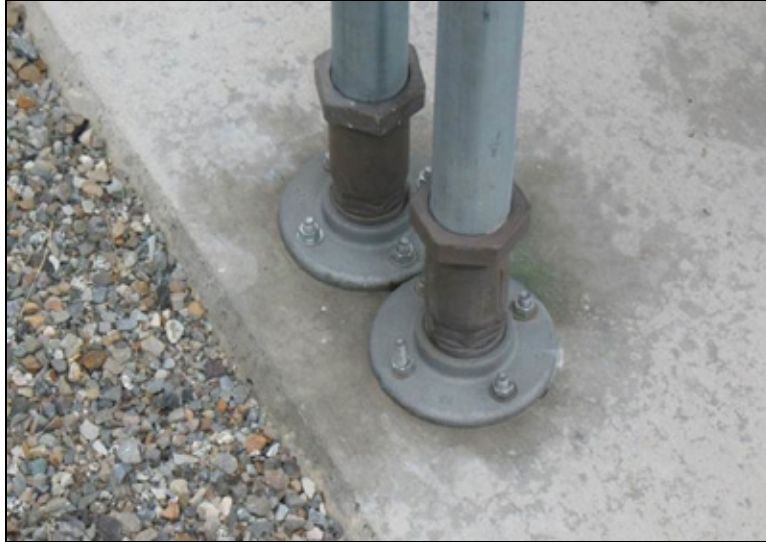
Figure 6-2. Two frangible connections
