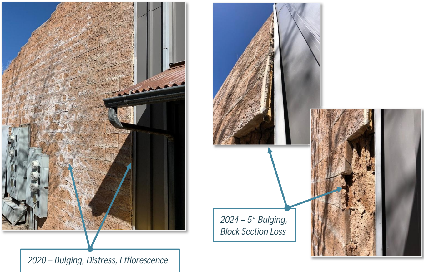
Figure 1: 2020 Wall Condition and 2024 Wall Condition
